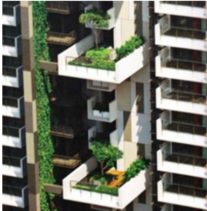
Figure 2. Newton Suite in Singapore. High-rise residential development incorporating exterior green walls, communal sky-rise gardens, and vertical greenery. [Source: Newman, 2014, p. 58]
