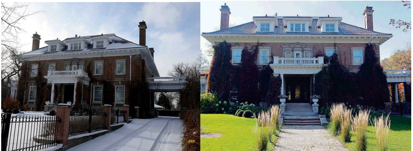
Figure 2: The Gordon House at 514 Wellington Crescent, shortly before it was demolished. (Source: George Penner/Manitoba Historical Society, Boris Minkevich/The Winnipeg Free Press)
