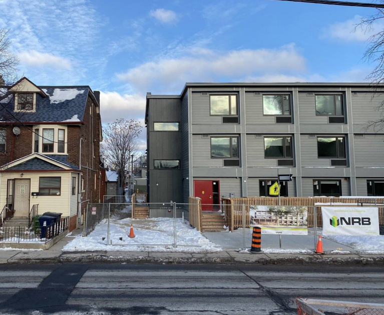
Modular at 321 Dovercourt Rd., Toronto
