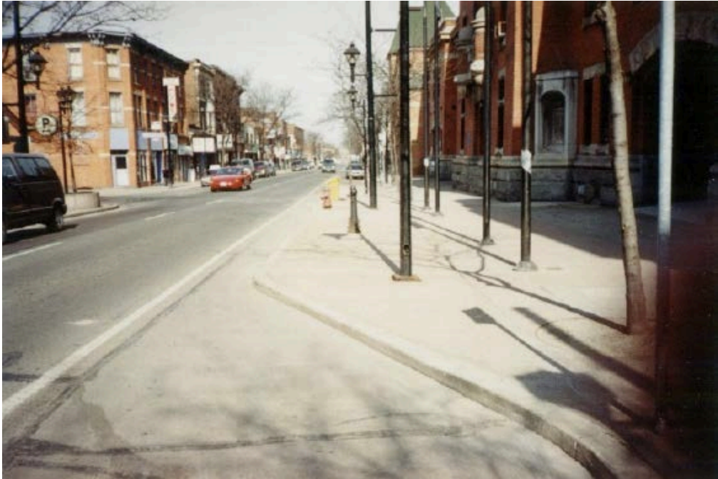
Figure 27: John Street North before conversion (IBI Group, n.d.)
