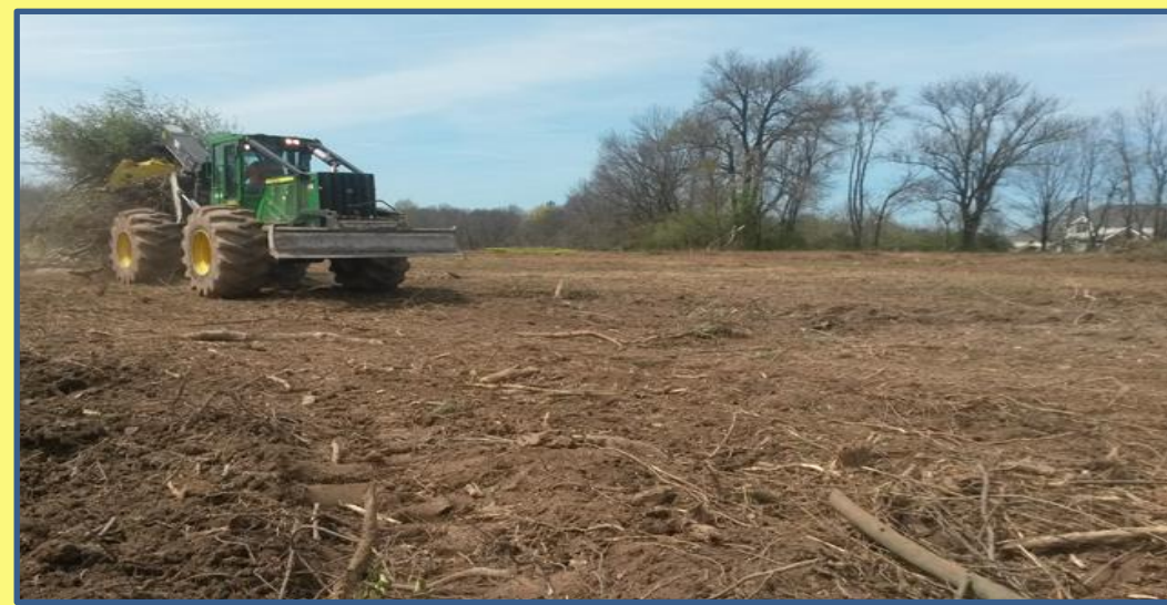
Brubacher.net, 2019, Site Clearing
